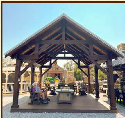
Appalachian - Hammer Beam
