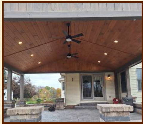
Ceiling under Rafters
